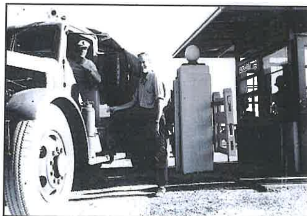
A truck load of fuel arrives at main gate
