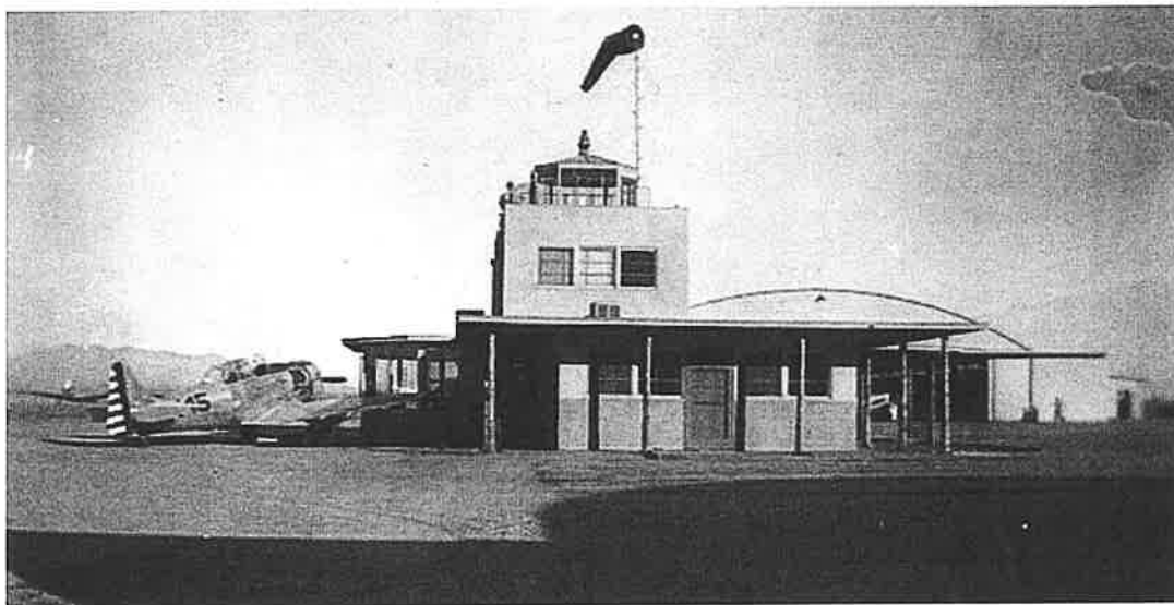
Control tower in late 1941
