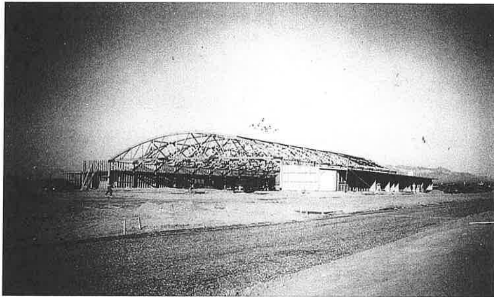
Partially built east hangar
